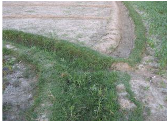
Fig.2 A root infested low height bank channel
