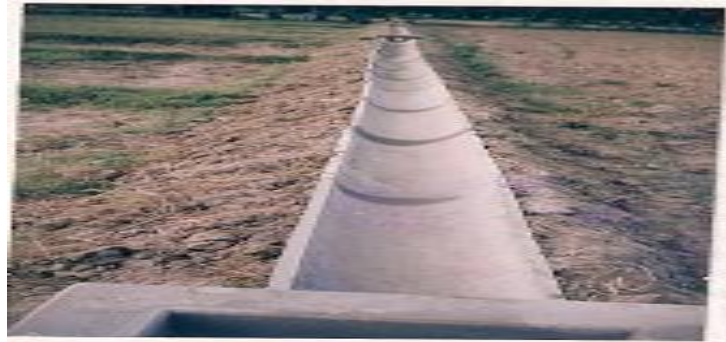
Fig. 10 A channel made of half round by jointing the sections
