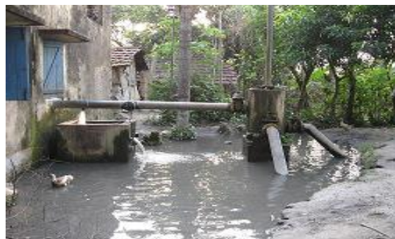
Fig. 7 Head end of a deep tube well irrigation channel system
